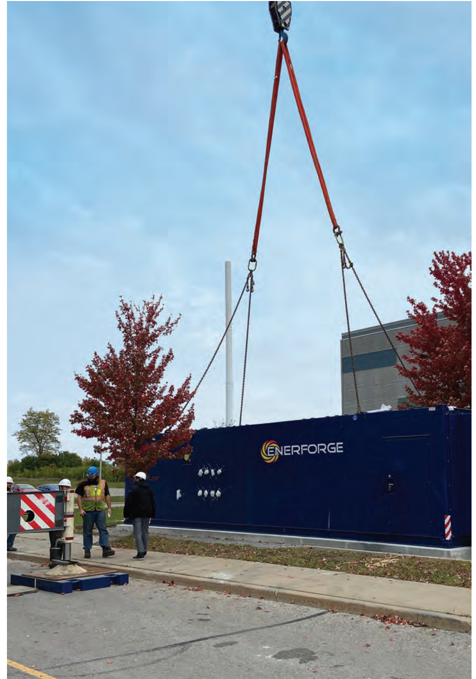
DELPARK CONTAINER ARRIVING FOR THE COMBINED HEAT AND POWER (CHP) INSTALLATION.
