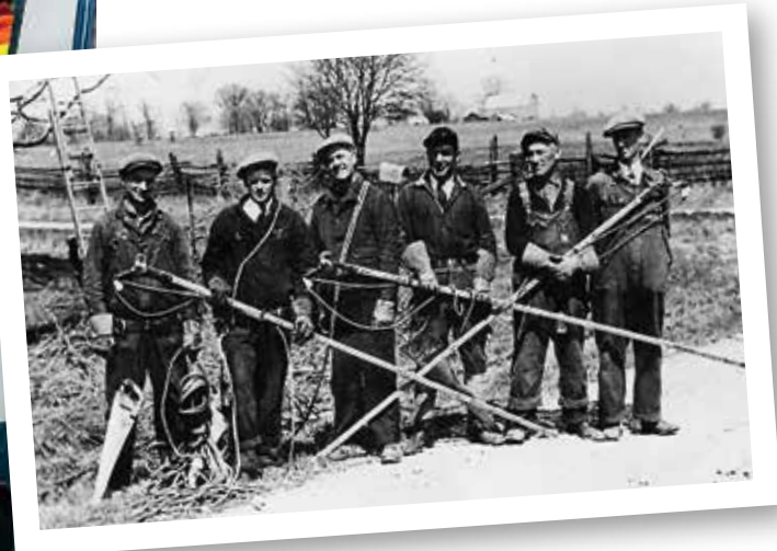
Line crew - 1945. Oshawa Power's full-time employee headcount stood at 85 in 2017.
