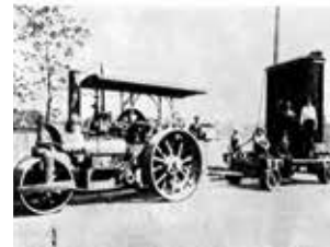
Crew moving a station transformer – 1919.
