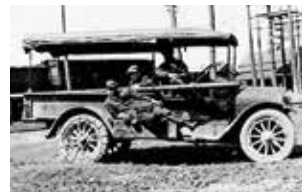
Construction truck equipped with chains for muddy roads.
