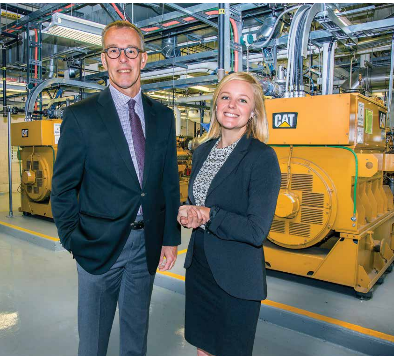
A team from OPUCN was instrumental in helping Lakeridge Health receive a $1.8 million incentive from the Province of Ontario for installing a 1.6 MW CHP plant at its Oshawa facility. Tim McHugh, Interim President & CEO, Lakeridge Health (left) and Janet Taylor, OPUCN's Manager of Conservation and Demand Management (right) are shown here in front of the plant.
